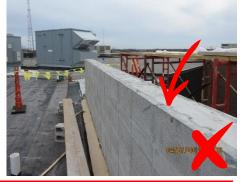
Wall is not protected at the top...even grouted solid walls must be protected
