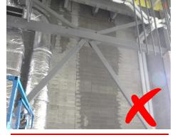
Water has entered from the top or is washing down the face of the interior CMU...this will cause the AVB to fail
