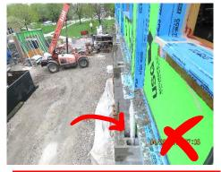
The wall as it is installed at the end of the day must be covered
